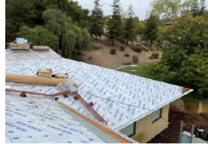
Cherry Hill Detox Roof Replacement
